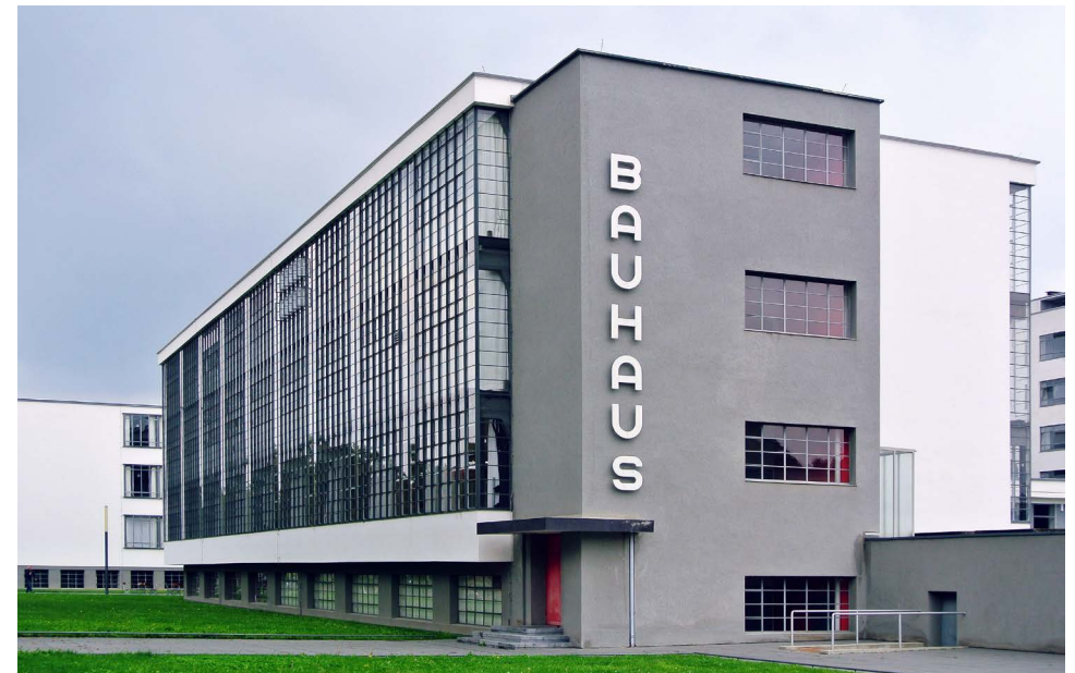
Gropius's Bauhaus Art school building in Dessau
