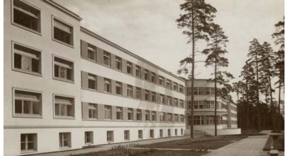
Tērvete. Sanatorium. 1930–1934. Designed by A. Klinklāvs and A. Kalniņš.
